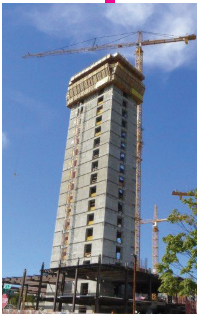
Fiber-reinforced concrete developed in part by UW-Madison engineers protects The Lincoln Square Expansion -- a 450-foot condo, hotel and office building rising in Bellevue, Washington -- against frequent earthquake activity. Credit: Courtesy Cary Kopczynski & Company
