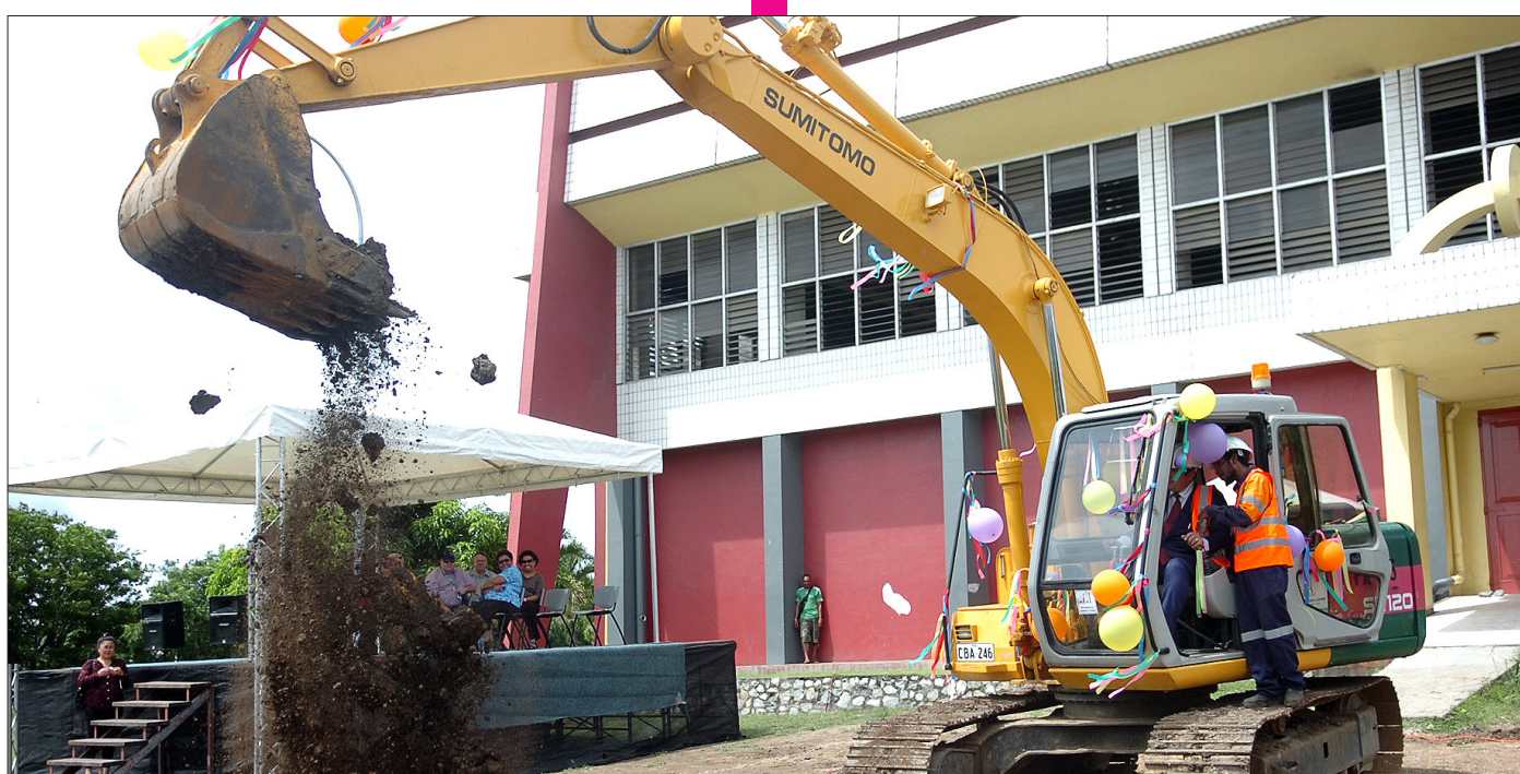
Groundbreaking: Work is launched on a city infrastructure project for the Pacific Games last year. Such building constructions were among the many infrastructure projects in Port Moresby last year as the country and the city experienced unprecedented growth.
