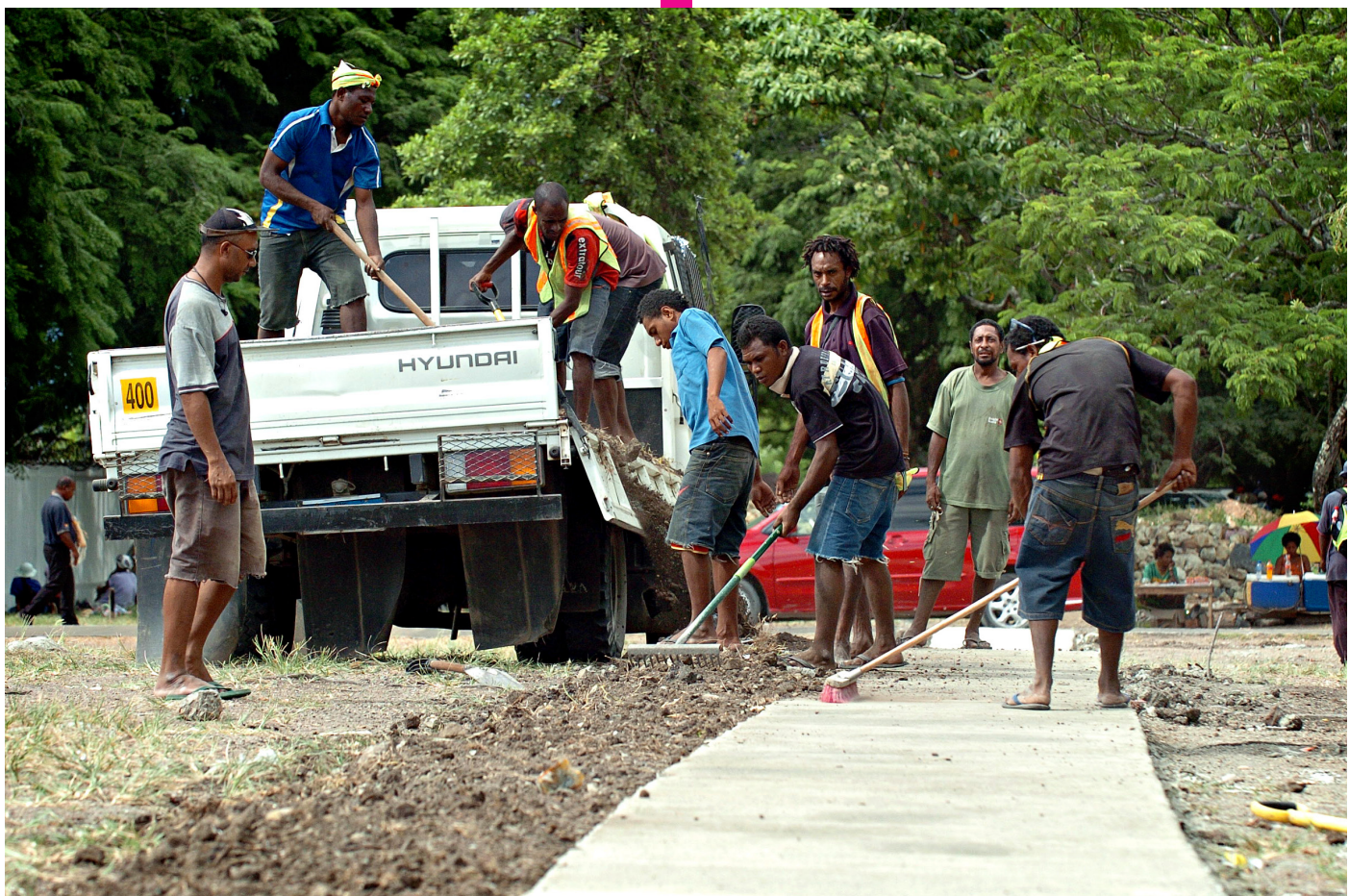
Contractors working on a civil construction work in Port Moresby. Even such minor engineering works must be certified by an engineer registered with IEPNG.
