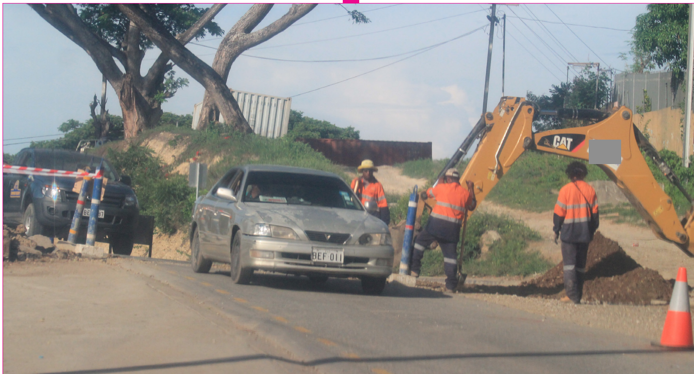
Contractors digging up a section of the newly-completed Two-Mile section of the Hubert Murray Highway in Port Moresby to fix service lines. The new software, when fully developed, could avoid such wastage and inconvenience
